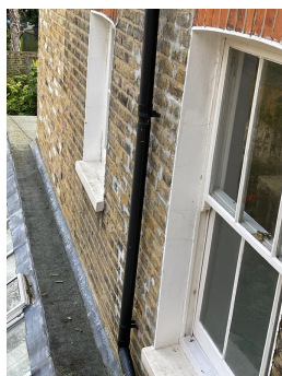
Photo 74 - Untidy pointing repairs
