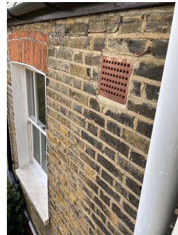
Photo 73 - Cracked pointing
