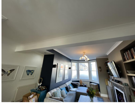
Photo 130 - Cross partition to living room removed
