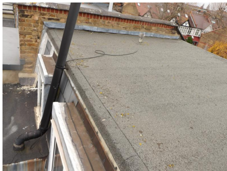
Photo 15 - Badly weathered felt
