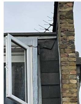
Photo 16 - Slipping slates to rear mansard
