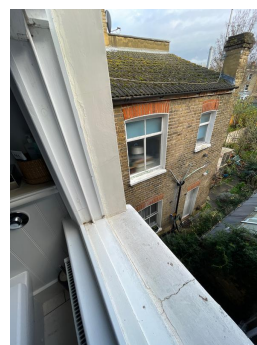
Photo 71 - Minor cracking to sill and window reveals
