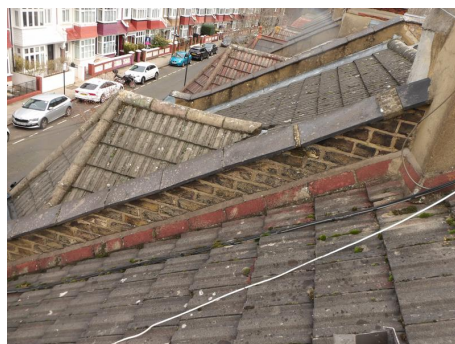
Photo 46 - Tillet fillets inadequate
