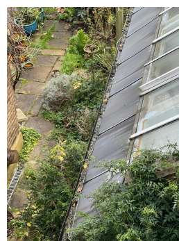
Photo 55 - Blocked gutters
