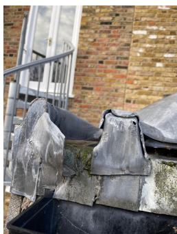
Photo 52 - Lead gutter
