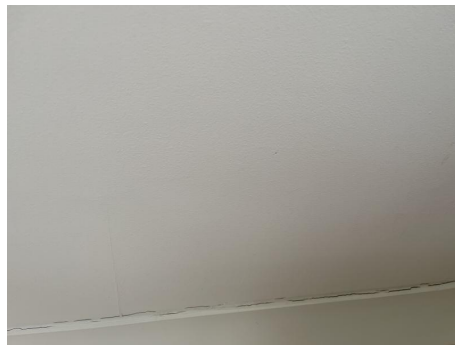
Photo 114 - Minor cracking
