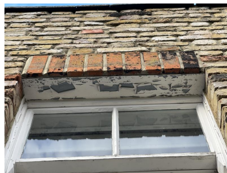
Photo 69 - Steel starting to peel and corrode
