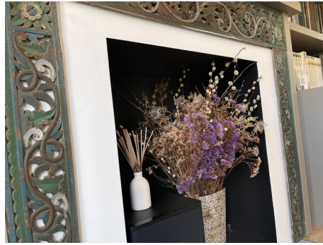
Photo 154 - No air vent to covered fireplace
