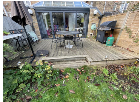
Photo 98 - Weathered timber decking
