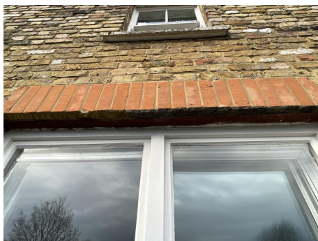
Photo 68 - Steel starting to corrode
