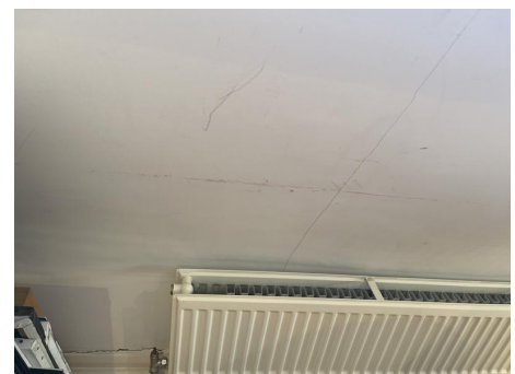
Photo 125 - Minor cracking and scuffing
