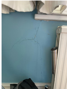
Photo 121 - Dampness and cracking to 1st floor rear bedroom
