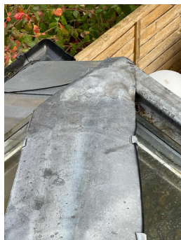
Photo 29 - Weathered and untidy felt
