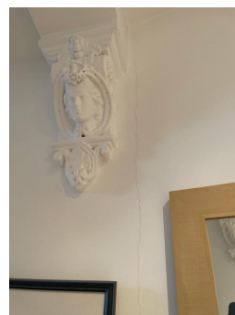
Photo 129 - Minor cracking
