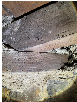
Photo 141 - Evidence of past wood boring insect infestation holes
