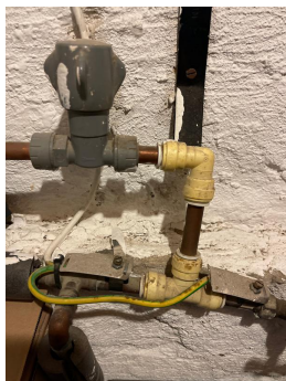
Photo 197 - Push fit connections
