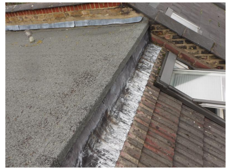
Photo 12 - Lead and felt badly weathered
