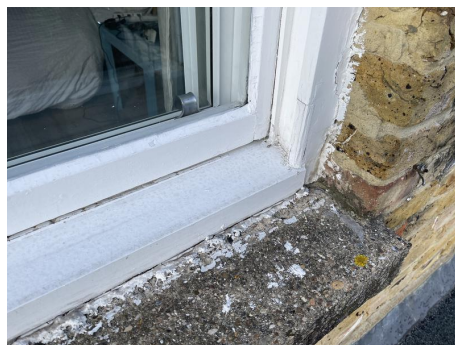
Photo 85 - Poor seals allowing damp ingress
