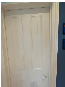
Photo 151 - Cracking to door
