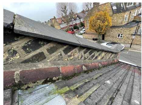
Photo 47 - Tillet fillets inadequate
