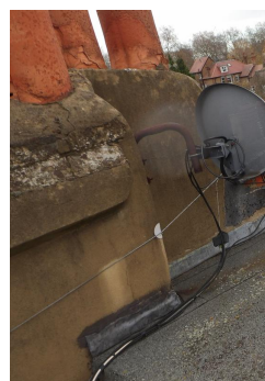
Photo 35 - Poor lead flashings
