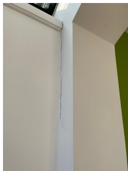
Photo 122 - Minor cracking
