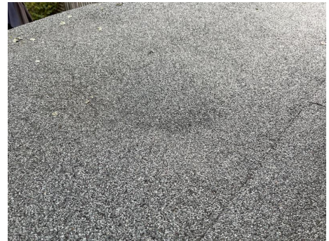
Photo 28 - Air pocket to felt
