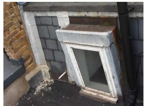
Photo 14 - Flashing tape repairs
