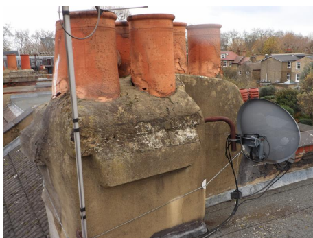
Photo 34 - Cracked and weathered render
