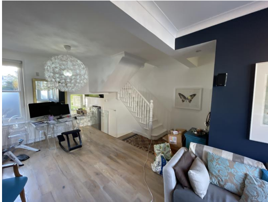
Open Plan layout with no protected fire escape route
